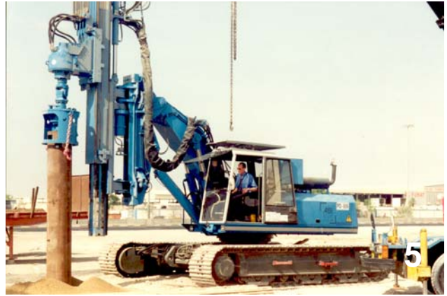
Picture 4: Positioning and drilling.
